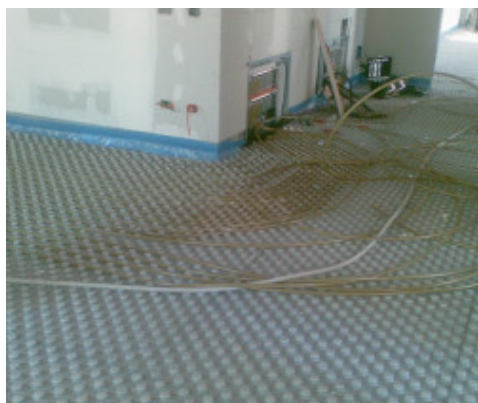
Preparation of the heating/cooling system
