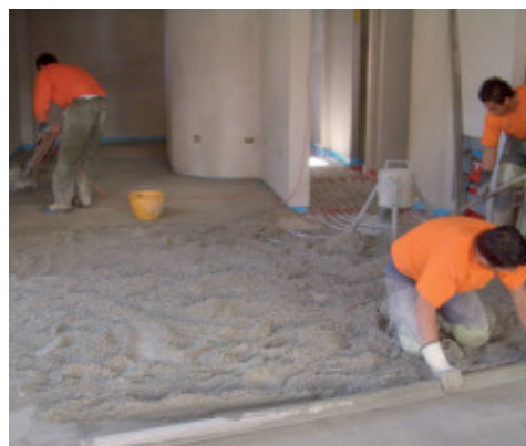
Spreading the mix with Mapescreed 704 admix
