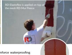
**RD-Mur Fleece** is micro-perforated and used to reinforce waterproofing systems and ensure the durability of the film. It reinforces the crack bridging abilities and will protect weaker parts from water ingress.
