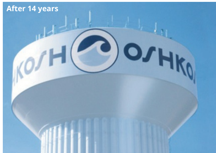
Oshkosh water tower PSX 700 was used to coat a water tower in Oshkosh, Wisconsin. Despite being situated directly next to Lake Michigan's moisture-abundant atmosphere, the tower still remains free of corrosion and mildew. It has also retained vibrant color and gloss, despite temperatures falling to minus 40°F during some winter months.
