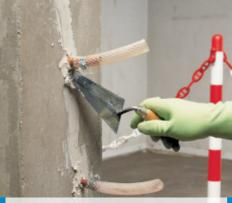
Fixing injection tubes and sealing cracks for structural consolidation
