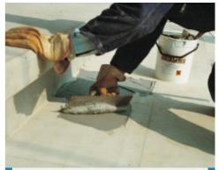
Application of Adesilex PG1 with a notched trowel for structural bonding of pre-fabricated steps
