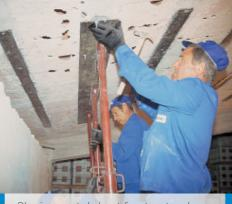
Placing metal sheet for structural reinforcement
