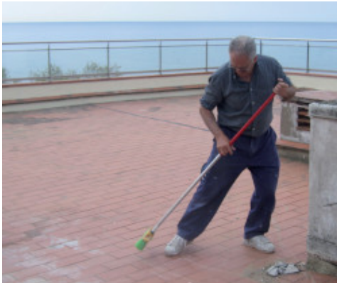
Cleaning a substrate before applying Aquaflex Roof
