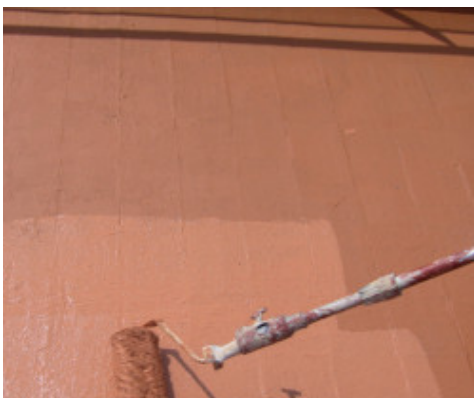
Application of Aquaflex Roof with a long-piled roller
