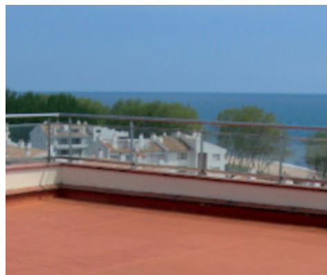
Paving slab waterproofed with Aquaflex Roof
