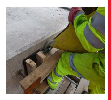
compressive strength of 60 MPa (at 20°C). The product shall be mixed and placed in accordance with the manufacturer's written instructions to a correctly placed substrate.
