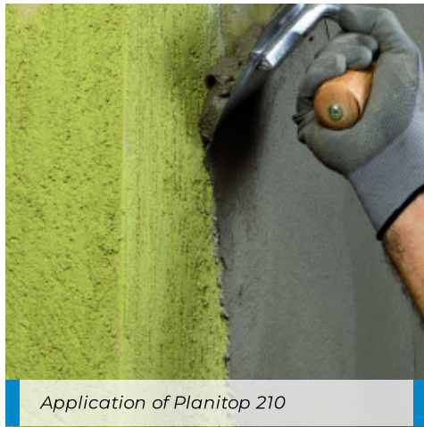
Floating the surface of Planitop 210
