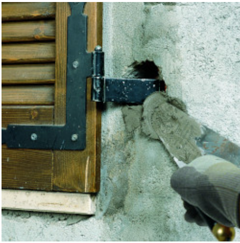
Fixing foundation bolts for windows using Lampocem
