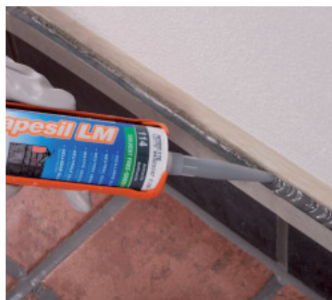
Sealing a fillet joint on natural stone
