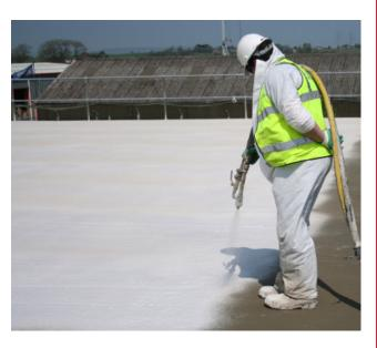
1mm thick coats (one coat white / one coat grey), to a correctly prepared substrate, in accordance with the manufacturer's written instructions.
