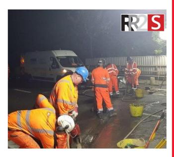
When used with a low water content, Patchroc 250 is designed for horizontal use, though it can be applied at gradients up to 2.5%.
