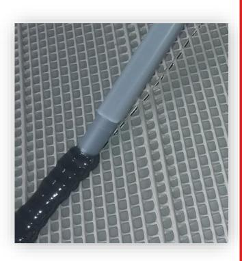
Halting application beyond the gel time will require a new static mixer to be installed before continuing.
