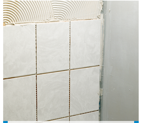
5. Apply grout and sealant
