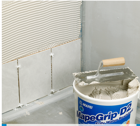
5. Tile using a suitable adhesive
