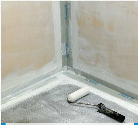
4. Apply a Mapegum WPS
