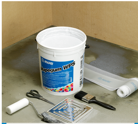
2. Prepare the tape for joints
