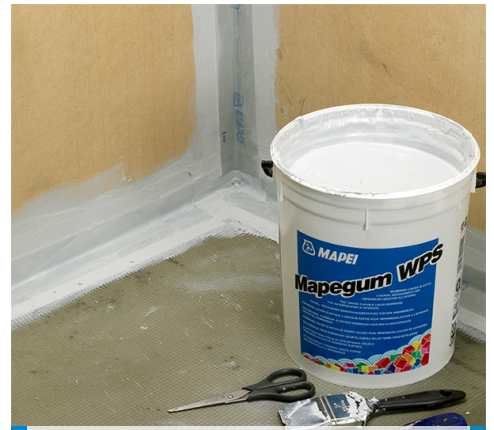
3. Apply the tape to the joints
