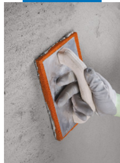
Tamping Planitop Smooth & Repair R2
