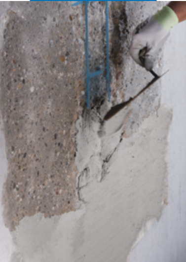
Application of Planitop Smooth & Repair R2 by trowel
