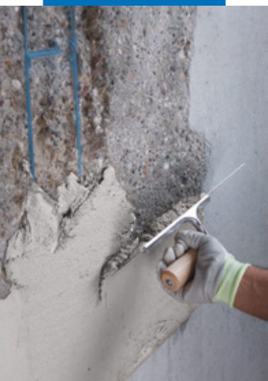
Application of Planitop Smooth & Repair R2 with a spatula
