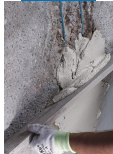
Smoothing of Planitop Smooth & Repair R2 with a straight edge
