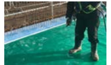
Testing of Proofex Total and Nitocote EP405
