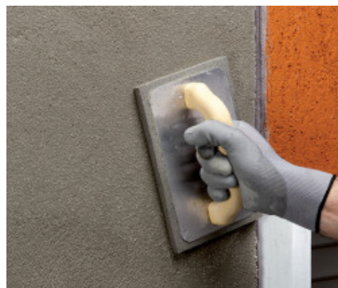
Floating the surface of Planitop 217
