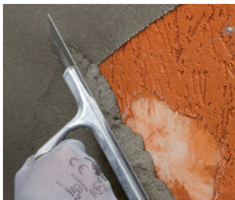
Application of Planitop 217
