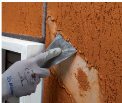
Removing all the plastic covering that has not adhered
