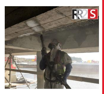
Renderoc DSR conforms to the requirements of Highways England, Standards for Highways, Specifications for Highways Works, clauses 5703, 5704, 5717 (Spray Applied Concrete Repair Materials) and 1704.5 (Control of Alkali-Silica Reaction).
